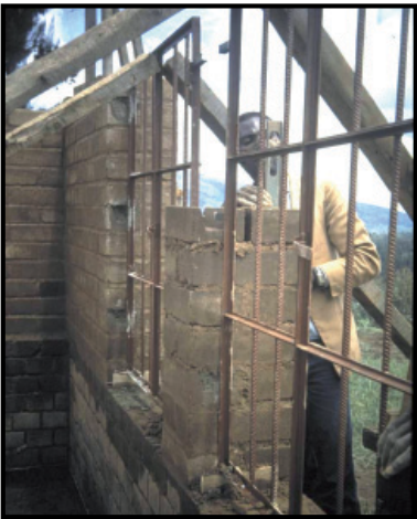
Sealing frames during brick work. Align the position of anchoring and U-shape blocks
